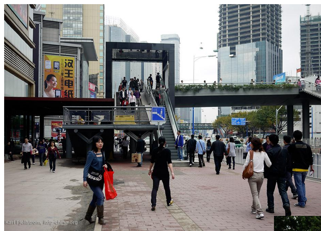
Integration of BRT station bridge & building, with double-tier bike parking under the bridge.
