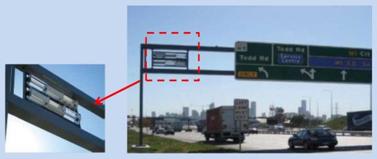
Figure 6-8: Windpods integrated directly to signage in Australia<sup>51</sup>
