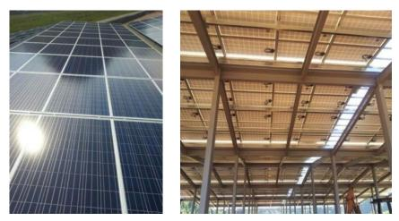
Figure 6-3: BIPV Rooftop installation with capacity 1.5 MW in Ipoh, Perak
