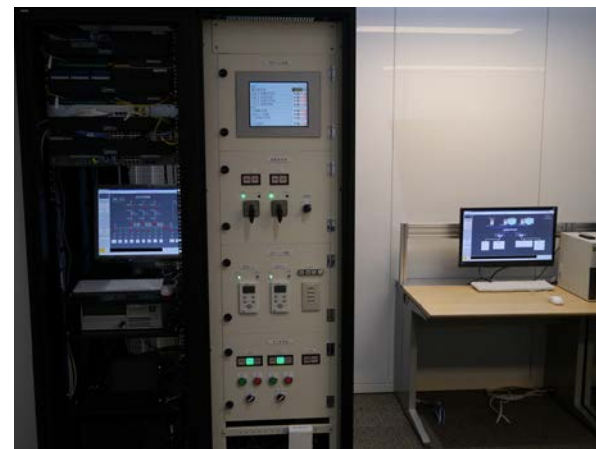
Building Plant II
