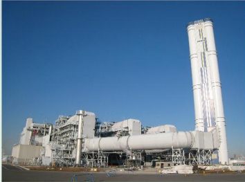
Integrated coal Gasification Combined Cycle (IGCC) Power Plants
