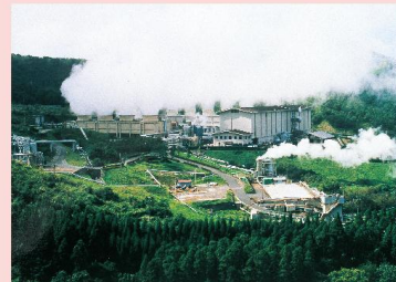
Geothermal Power Plants
