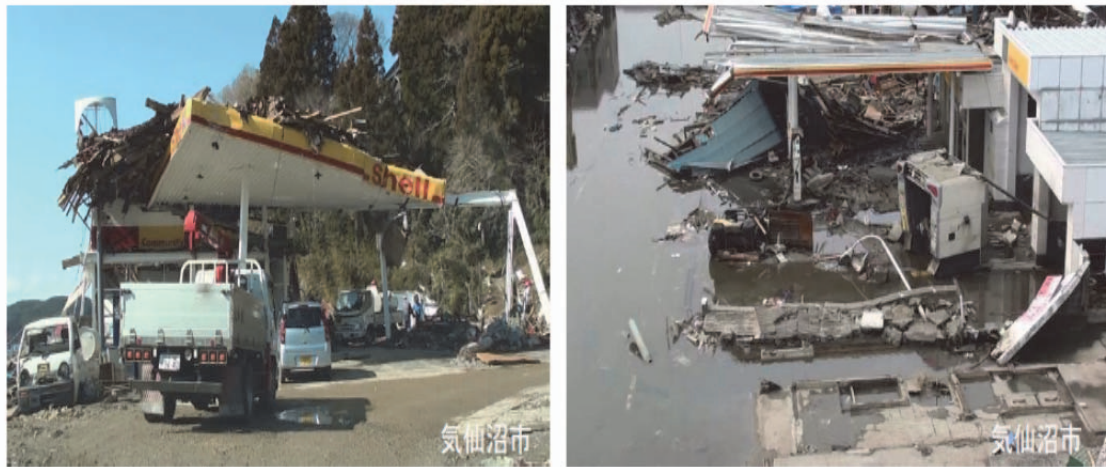
Figure 3 (Damaged service station in Kesenuma City)
