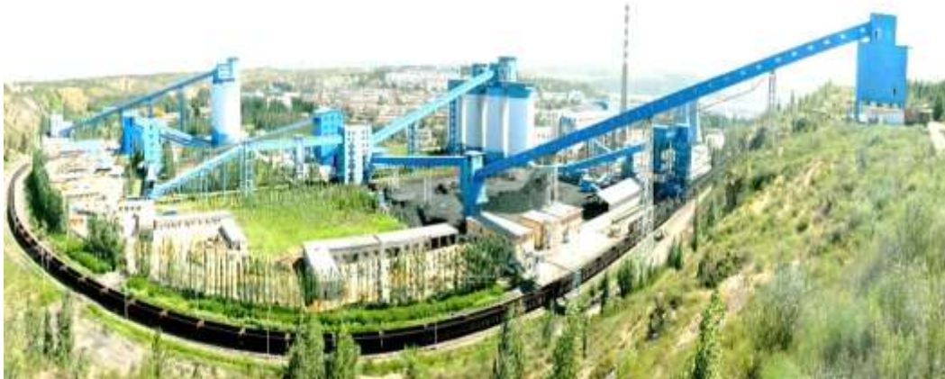
Shangwan Coal mine in Shandong
