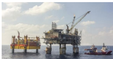
The Malampaya Gas Platform Offshore of Palawan Source: Shell Philippines Exploration, B.V.
