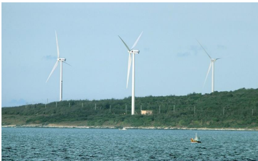
Figure 1.19: PVN's 6 MW wind-diesel hybrid system in Phu Quy island, Viet Nam
