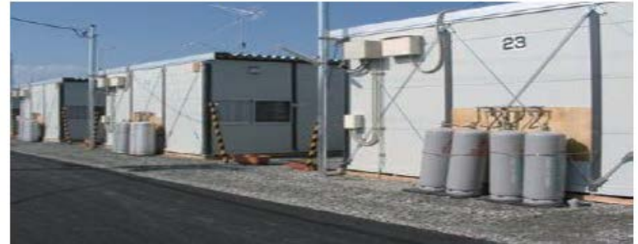
LPG cylinders at a temporary housing project
