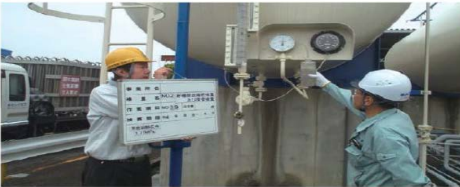
Storage tank airtightness test Storage tanks are inspected for gas leak.
