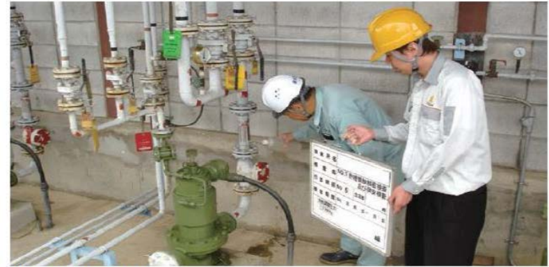
Piping airtightness test Piping sections are inspected for gas leak.
