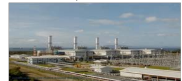
1,000 MW Sta. Rita First Gen/ IPP
