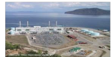
1,200 MW Ilijan Power Plant NPC IPP(KEPCO)
