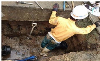
Gas pipe repair
