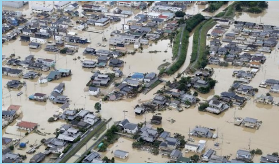
Flood caused by downpour in west Japan
