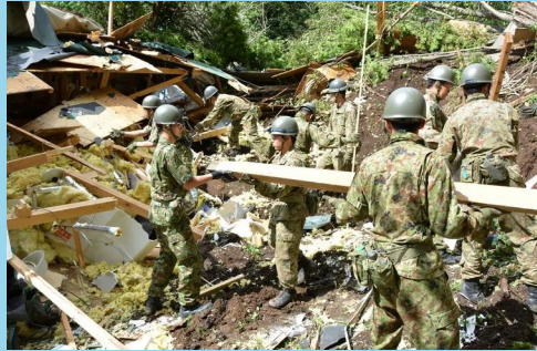
House collapsed by earthquake in Hokkaido
